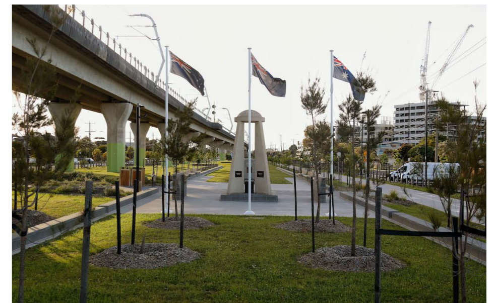
QB55- Cenotaph, Clayton, VIC Demonstrates a successful memorial relocation undertaken in consultation with stakeholders which is well-integrated into the design of new public realm. Image: Level Crossing Removal Project.
