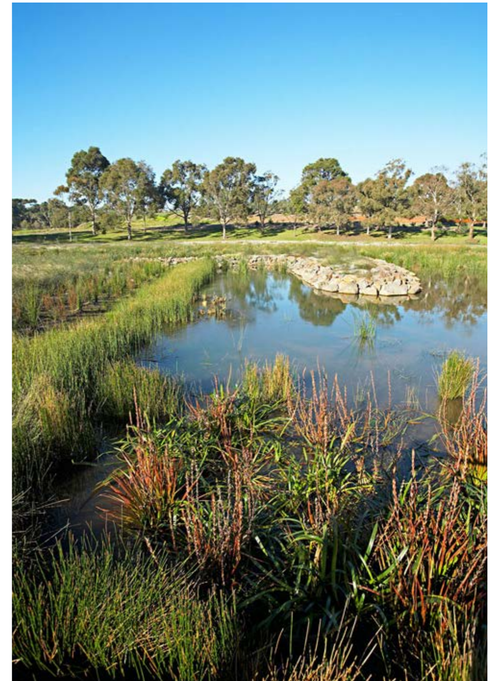
QB26 - Royal Park Wetland, Melbourne, VIC Demonstrates attractive stormwater harvesting and water quality treatment in a constructed wetland. Design: Rush Wright Associates. Photographer: Michael Wright
