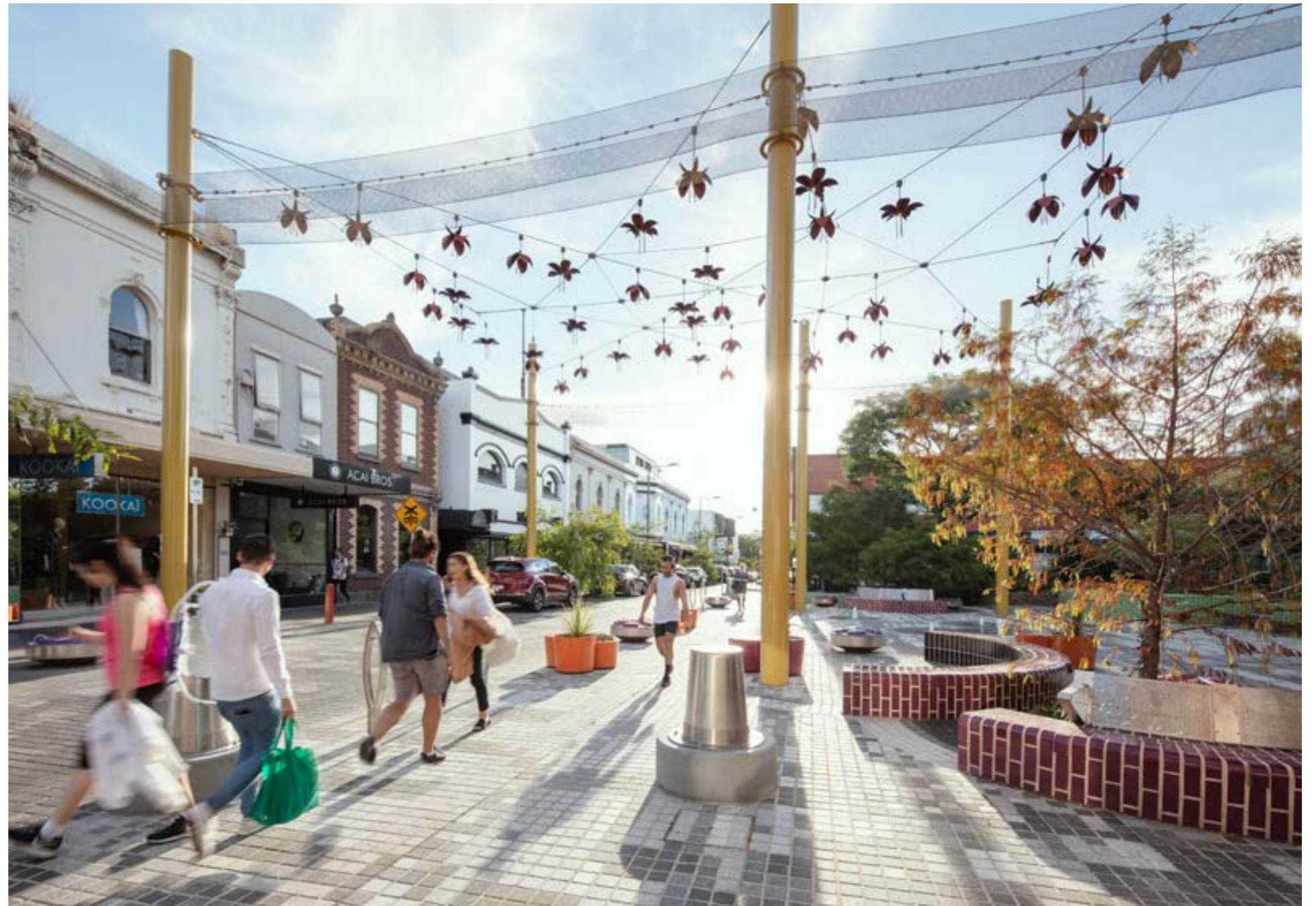
QB43- Greville Street Precinct, Prahran, VIC Demonstrates well-executed public realm using the selections of materials and arrangement of public realm elements to support transitions between pedestrian and shared mode spaces. Design: Rush Wright Associates. Photographer: John Gollings.
