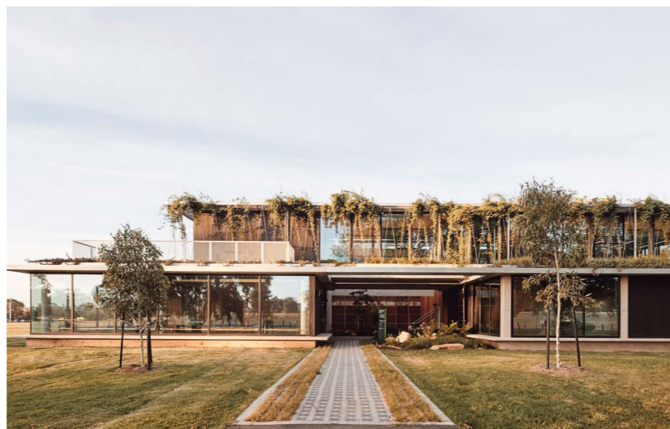
QB08 - Albert Park Office and Depot, Melbourne, VIC Demonstrates a well-designed building that sits comfortably in its context and contributes to positive place outcomes. Design: Archier, Harrison and White. Photographer: Peter Bennetts.
