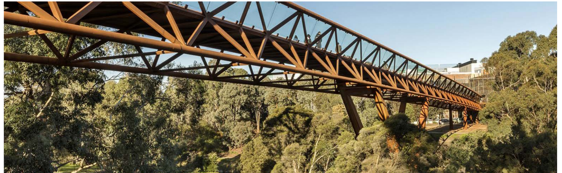
QB44 - Burwood Link, Burwood, VIC Demonstrates a structurally expressive bridge structure that is contextually sensitive. Design: watsonarchitecture+design. Photographer: Lisbeth Grossmann.
