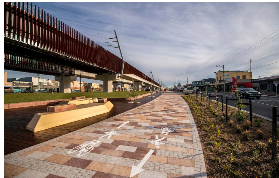
QB48 - Carrum station, VIC Demonstrates the use of public realm materials to define space allocation for different transport modes. Design: Rush Wright Associates. Image: Level Crossing Removal Project.
